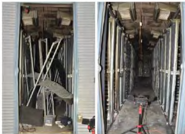
Figure 8 Additional view of debris and damage to the rear door, HVAC systems, and the container
