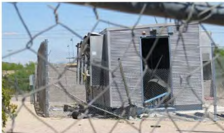
Figure 8 Additional view of debris and damage to the rear door, HVAC systems, and the container
